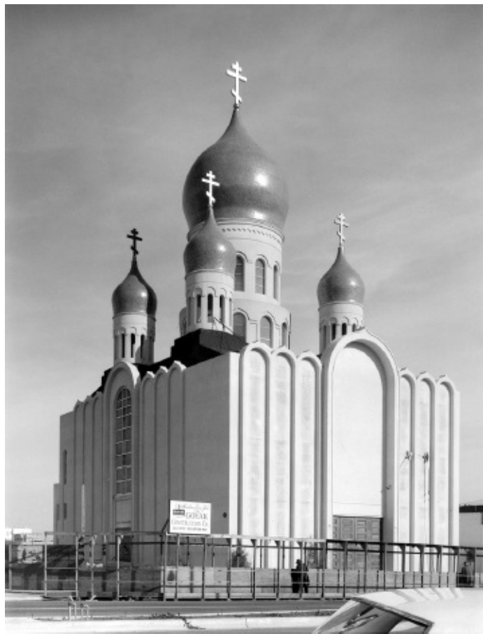
The new “Joy of All Who Sorrow” Cathedral on Geary Boulevard in San Francisco, while construction on it was being completed.
